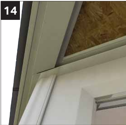
14 External ship lap cladding edge channel detail.
