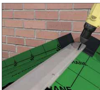
Fixing ridge under capping into tile stop
