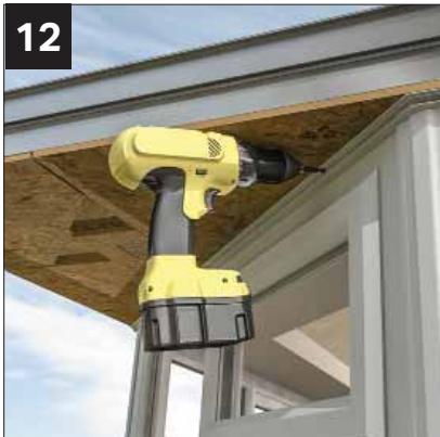
12 Fit external soffit channeling.
