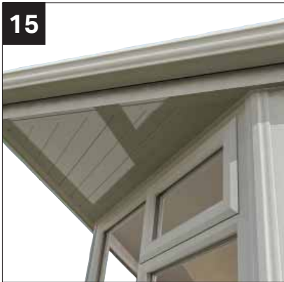
15 Cut and fit ship lap to suit.
