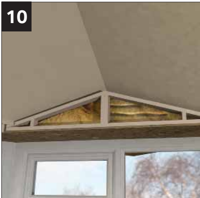
10 Insulate void with mineral wool.
