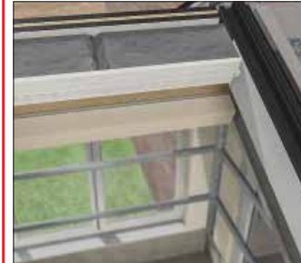
Fitting upper plasterboard trim
