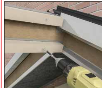
Fitting of the timber ridge battens
