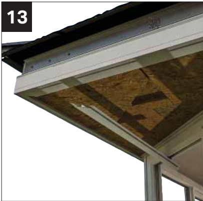
13 Fit external ship lap cladding edge channel.
