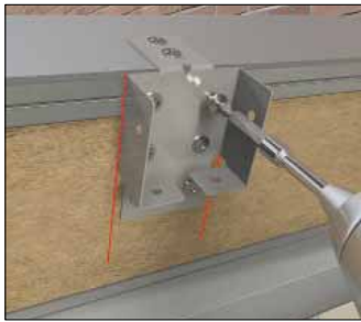
Fixing glazing bar shoes to ridge section
