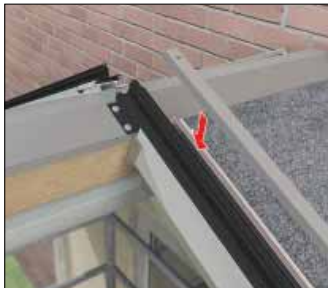
Fixing glazing bar to ridge
