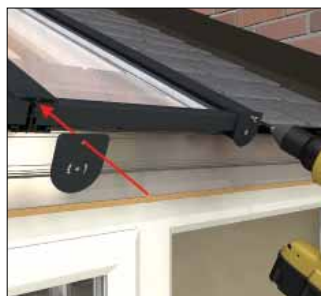
Fixing glazing bar end caps
