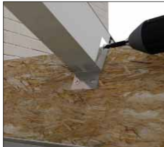
Fixing glazing bar at box beam shoe
