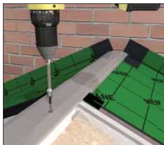
Fixing ridge under capping central
