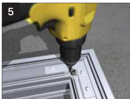
If supplied, fasten to each corner the tie bar drop rod fixing bracket to the underside of the lantern eaves beam.
