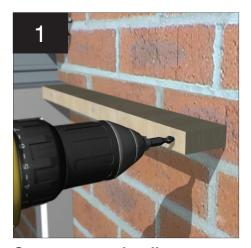
**Gutter return detail** - If the gutter returns along the host wall, a timber section is required to support the lower section of the cornice. Ensure the treated timber baton (49mm x 20mm) is level, then fix into position.
