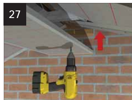
Fit the ridge board as described on page 39.
