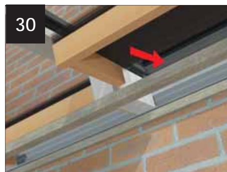
Slide remaining modesty panels into position, ensure that the batten on the screen is set 6mm back and screw fix to secure.
