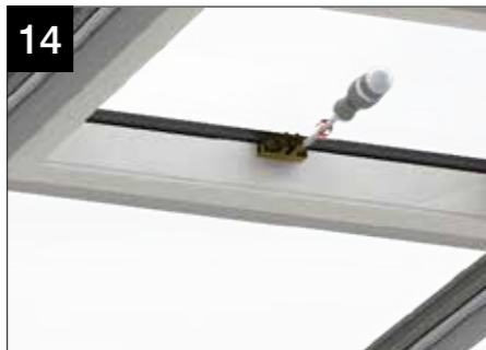
14 Using the screws provided attach the spindle bracket to the sash bracket (already attached to vent sash) taking care not to damage the glazed unit.
