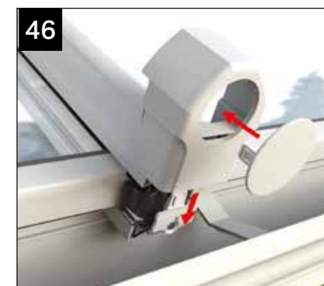
46 If you haven't fitted already, attach end cap fixing blocks - These arrive attached to the end caps. Fit the glazing bar end caps by sliding onto the fixing blocks. Push fit the insert into the end cap.
