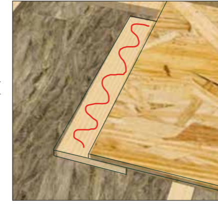
You may encounter panel joints that cannot be supported by either the tongue and groove connection or by a 2x2 firing. In this instance, 6x1 timber is provided to support these joints. Cut the timber to the length required, glue one side and position underneath joint. Lay next OSB in position and nail through to secure.
