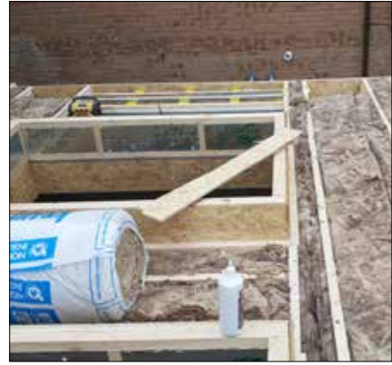
First, fill up the gap between the firings using the insulation before the deck is fitted.
