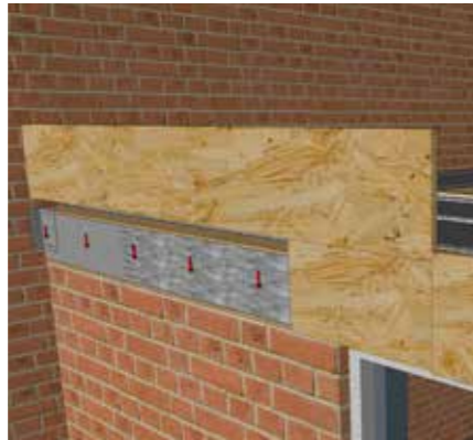
Place OSB fascia 1b, overlapping the first fascia.
