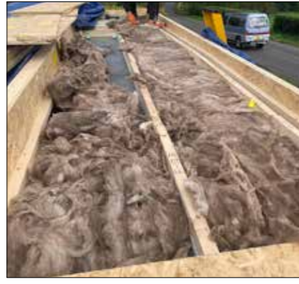
First, fill up the gap between the firings using the insulation before the deck is fitted.
