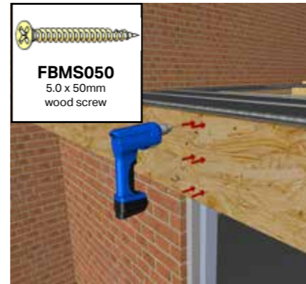
Once aligned, fix through the joint of the two OSB fascia using 6 fixings and then continue to fix into the beam using 3 FBMS050 fixings per 400mm centres.
