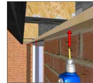
Soffit batten to underside of fin
