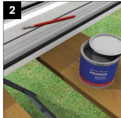
2 Ensure the surface is dry – apply a thin primer coat using a fine brush.
