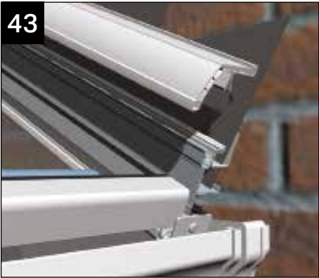
Ensure the rain baffle upper leg is lifted prior to fitting the top cappings.
