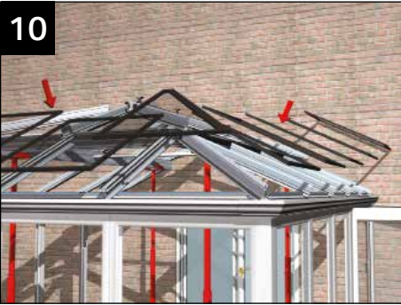
Glaze the lower pagoda roof fully.
