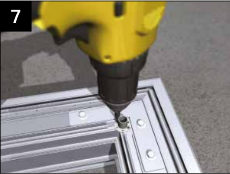
If supplied, fasten to each corner the tie bar drop rod fixing bracket to the underside of the pagoda eaves beam.
