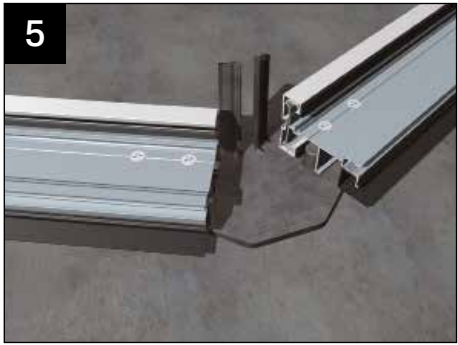
Take the second starter bar and similarly offer this onto the ridge hanger/compression plate assembly. Lift the whole "A" frame assembly and get ready to install it in its final position.
