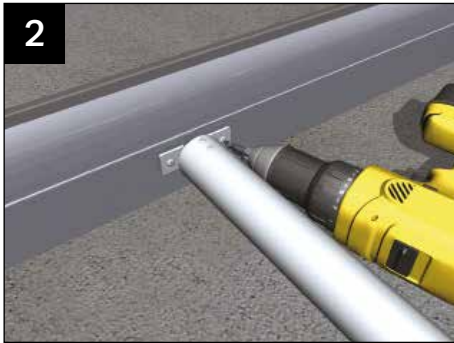
Attach the strut at the mid point of the long sides.
