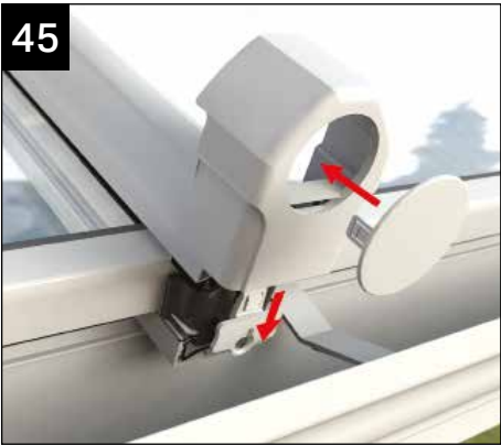
If you haven't fitted already, attach end cap fixing blocks - These arrive attached to the end caps. Fit the glazing bar end caps by sliding onto the fixing blocks. Push fit the insert into the end cap.
