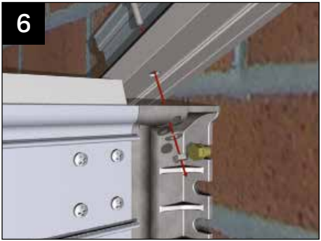
Attach the starter bar using the nut, bolt and spring washer (included in the kit) to the eaves structural moulding. Finger tighten the nut to temporarily allow the assembly to hang.
