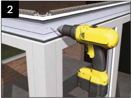
Two pilot holes already exist in the next piece of eaves beam – drill two more at 4.5mm diameter through the eaves beam and the cleat and then securely fit the four M5 x 12mm tapite screws.
