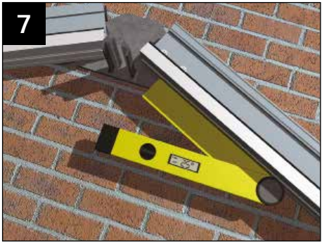
To set the ridge use an "angle fix" - check the starter bars are at the correct pitch. Chalk/pencil a line on to the wall to mark the pitch line.
