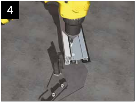
On the ground, away from the conservatory, offer up the first pre-drilled starter bar. Onto the ridge hanger plate fasten using the set screws provided - do not over tighten.
