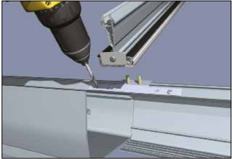
180° INLINE EAVES TO BOX GUTTER JOINT Place the inline cleat (SES003) over the butt joint. Offer the glazing bar on to the bolts, align and secure. Once in position fix the cleat down with the two fixings supplied (UZBGF001-D). Note: Only two of the four holes are used.
